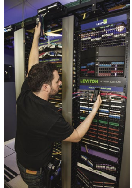
Reading FiberChek probe results on a smartphone
