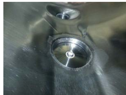
Figure 2 VS3000E probe attached to Research White Wine Fermentation tank inside tank view.
